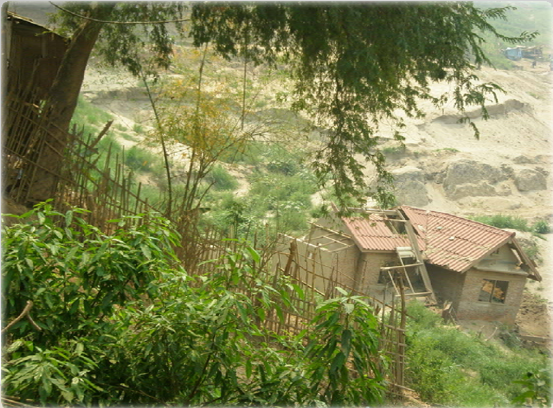
Houses destroyed in the flood Taken from the temple'09,3
