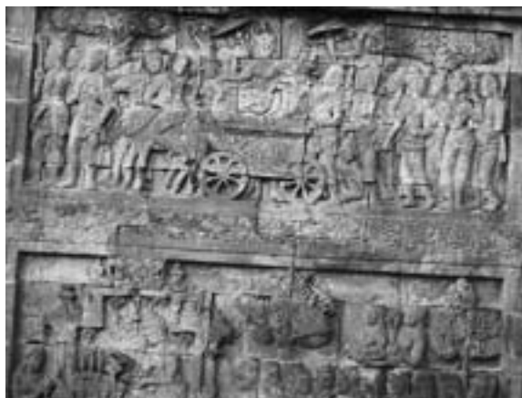
Figure 3. One of the deteriorated narrative panels on Lalitavistara
