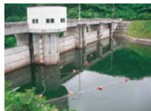
■ Field experiment at Sounoseki-dam (Miyagi Pref.)
