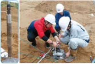
■ Subsurface soil strength measurement using a miniature borehole testing tool
