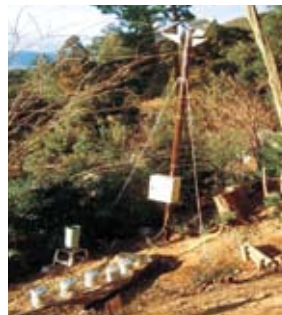
■ Long-term measurement implemented at Kiyomizu Temple using the slope disaster prevention monitoring system. A tensiometer that measures the water volume of the surface layer of the slope is the center of the sensor.
