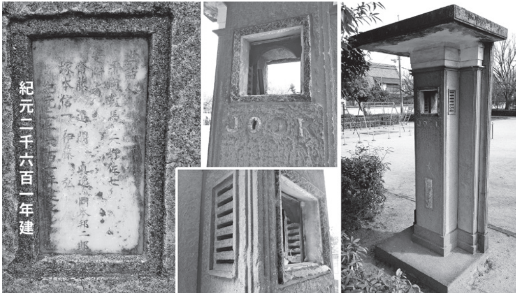
Figure 6: This unusually-shaped, non-symmetric tower still retains the JOOK call-sign and a plaque marking its establishment 1940.
