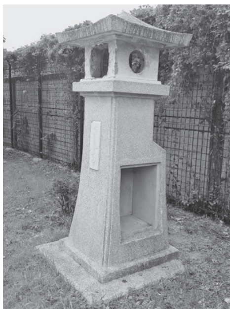
Figure 7: The Tachibana-jidō Park tower, shows few of its original features after restoration.
