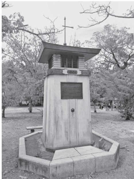
Figure 3: Radio tower in Maruyama Park, Kyoto.
