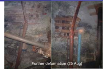
Photo 5. Considerable roof deformation associated with mining advance.
