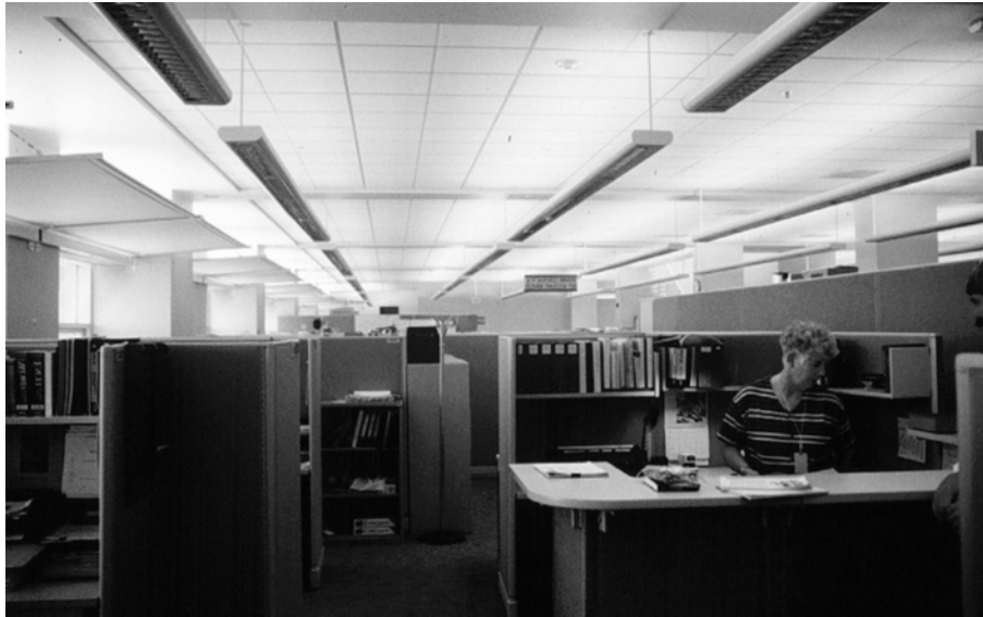
光の棚を取り付けたオフィス室内 Interior of office equipped with light-shelves (IEA, 2000, Daylight in Buildings)
