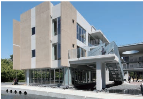
BKC Tricea: New Science & Engineering Building II (in use from May 2014)
