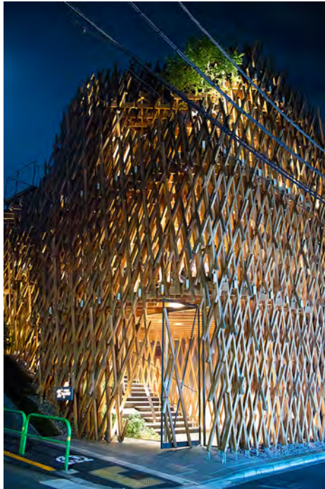
Figure 9: SunnyHills cake shop in Minami-Aoyama, Tokyo, designed by Kengo Kuma in 2013. The building's shape is inspired by a pineapple.
