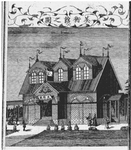
Figure 1: An engraving from an unknown artisan of a building from the First National Industrial Exhibition ( Naikoku Kangyō Hakurankai ), first held in 1877, Ueno, Tokyo.
